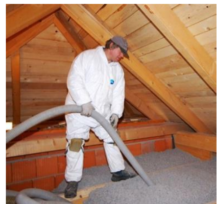
Figure 2: Cellulose insulation in open attics
