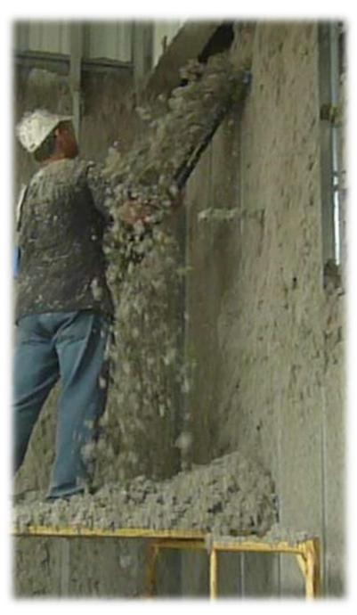
Our **Cool Tools** are important devices used to remove excess wall spray insulation (flush) with wall studs, allowing for easy installation of drywall. The 'wall scrubbing' process must be fast and easy, resulting in a clean surface that will compliment the spray process.
